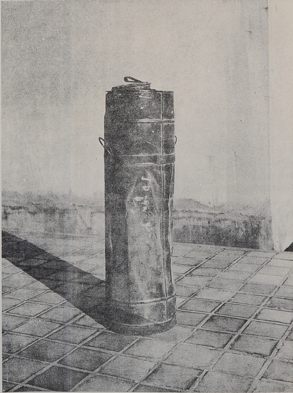
7. Crushed blue - print container from Hiroshima. Distance 5000ft., peak pressure 3.8 p.s.i.
